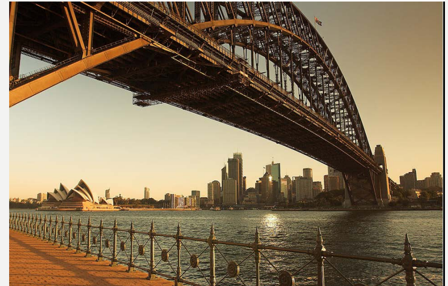
↑ The Harbour Bridge
