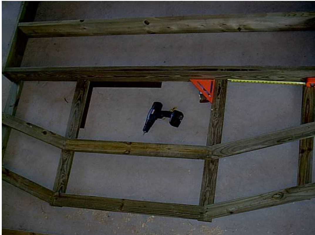
Figure 4 I used the frame as a stop for the bottoms of the guard rail.
