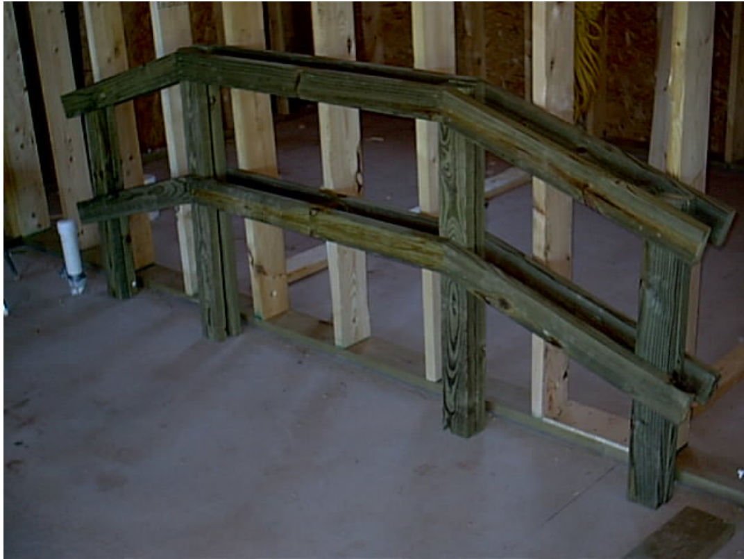
Figure 5 The two guard rail assemblies should match when placed back to back.
