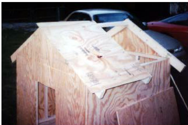
Complete framing before the application of plywood. Note crowbar.
