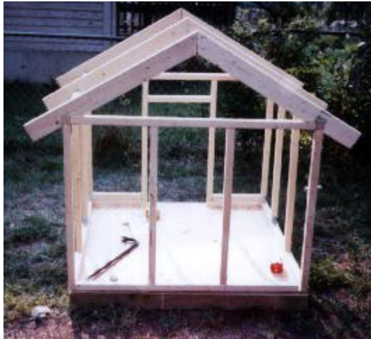
Complete framing before the application of plywood. Note crowbar.
