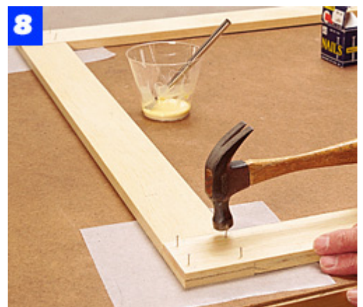
Spread glue on both surfaces of the rear frame's half-lap joints. Nail the pieces together from both directions.
