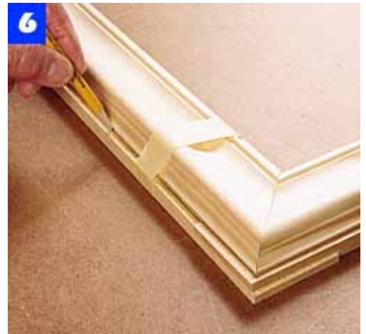
Tape the face and rear frames together with an equal reveal on all sides. Mark the rear frame with a pencil.
