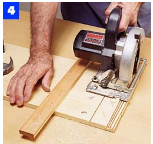
Nail a cleat across the rear frame pieces. Cut the shoulder, and make parallel cuts with a circular saw.
