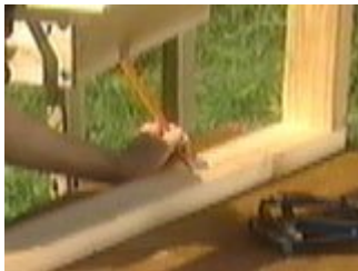
Mark the centre of the frame along the inside
