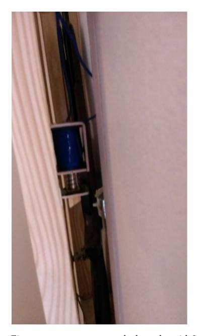
Figure out a way to attach the solenoid, I used a small steel strap with holes in it to screw the solenoid to the door.(also used epoxy)
