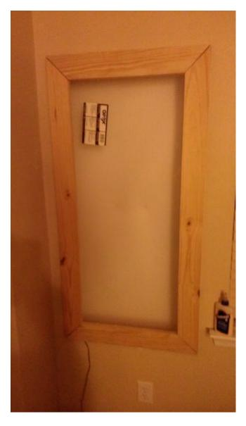
I used 1x4's to make a 2' by 4' door using a table saw I cut a groove into the side of the 1x4 to hold the mirror then cut a 45 degree angle on the ends of the 1x4's then assembled. Then add cabinet hinges.
