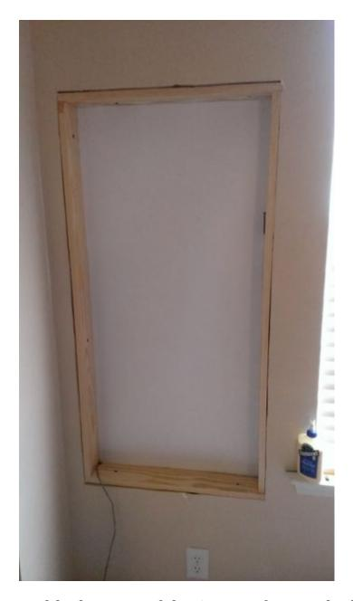
Build a box out of the 1x4s to fit into the hole since the box is going to be slid out to the edge of the drywall there is going to be a 1/2 gap behind the box and the other side of the wall.
