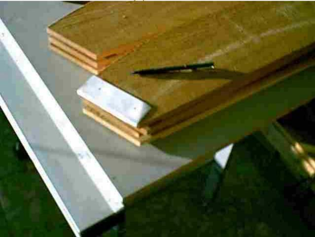
Drill the holes for the size of screws you'll be using and countersink them so the screws will be flush. I used 2", #6, flathead, exterior screws. Be sure and keep the matching segments together because each side is a mirror image and the segments need to match.
