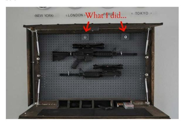
I first decided where I wanted my case to be placed. I then determined where the studs where on the wall that I was mounting my case. As you can see my lag screws are not centered. This is because I placed the lag screws according to the stud placement.
