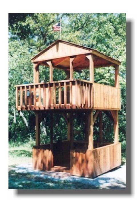
**Step1:** Frame 1st and 2nd floor system following diagrams shown. Use 2x6x8' pressure treated lumber and measure to have outside to outside dimensions exactly 8' x 8' on first floor, and 8' x 10' for the 2nd floor.
