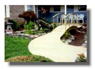
The bridge is made of two pressure treated 2x12 stringers. Determine the arch needed based on your conditions. You can use a string with a tack at one end and a pencil at the other as a compass to draw the arch. A note of caution...it's easy to have an arch that is too steep. It's better to have a shallow bridge rise that is safe to traverse in any weather. The one pictured above is the maximum rise you would want.
