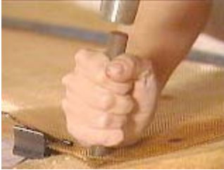
Place the punch over the mark and strike it with a hammer until it has pierced all layers of screen
