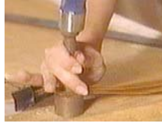
Insert the setting tool and strike with a hammer
