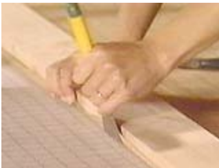
Use a putty knife and the straight edge to bend the screen up
