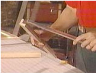
Build a 90 degree wooden jig
